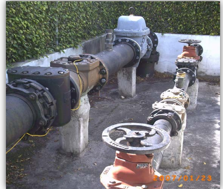
Imported water supply flowmeters
