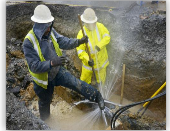
Temporary “broomstick” repair of a blown ferrule
