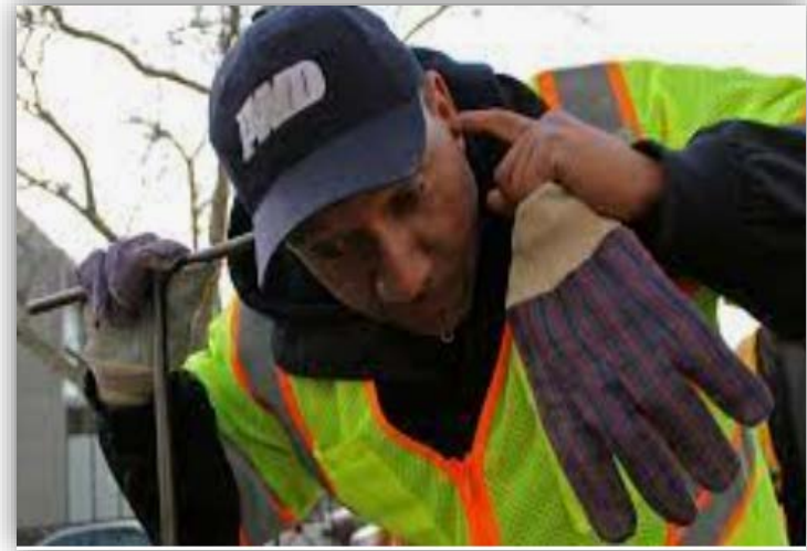
Sounding a valve key touching a valve
