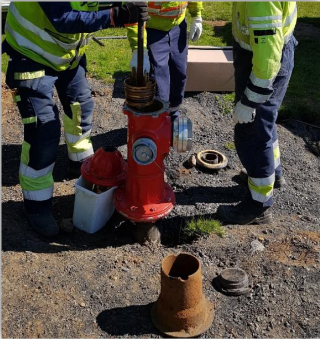
Hydrophone retrofitted to fire hydrant base Courtesy of Digital Water Solutions
