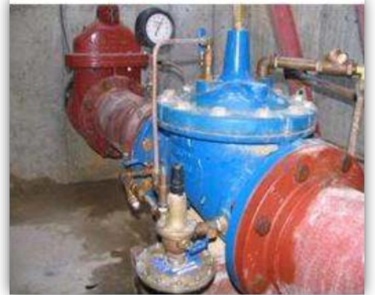
Pressure Reducing Valve (PRV)
