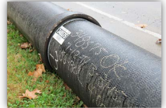
Replacement ductile iron pipe ready for installation
