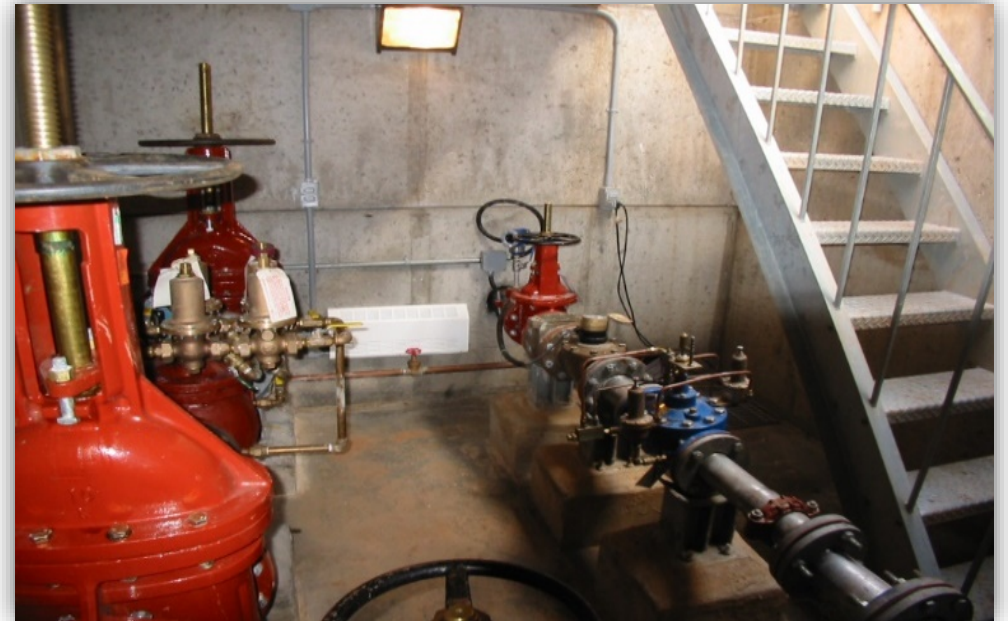
Pressure Reducing Valves for pressure management in Halifax, Nova Scotia, Canada
