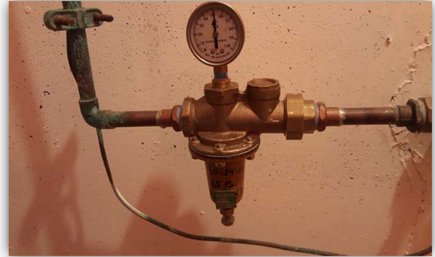
Pressure Reducing Valve (PRV) installed on a residential customer service line
